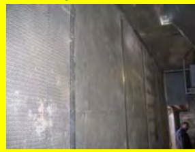
Wall & ceiling insulation
